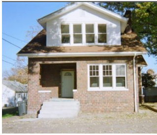
Oxford House-West Washington Huntington, West Virginia
