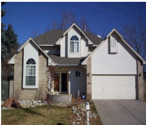
Oxford House - Kenton 1488 S Kenton Street Aurora, CO 80012-4120 7 W • Established June 1, 2006
