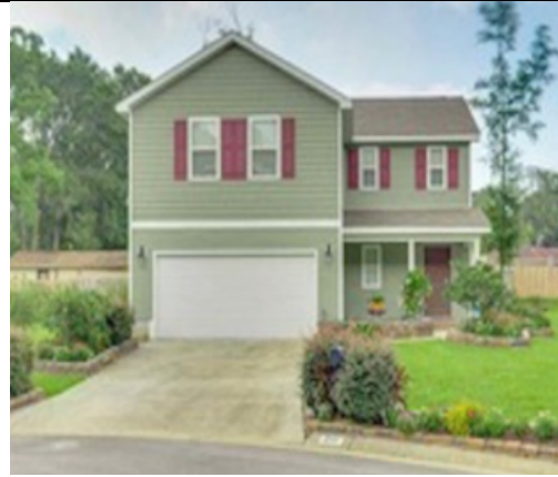
Oxford House - Waltham 2111 Waltham St. Pensacola, FL 32505 9 M • Established December 1, 2019
